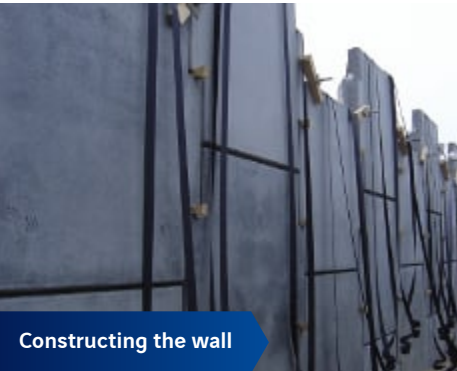
Installing the reinforcements
