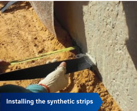
Installing the reinforcements
