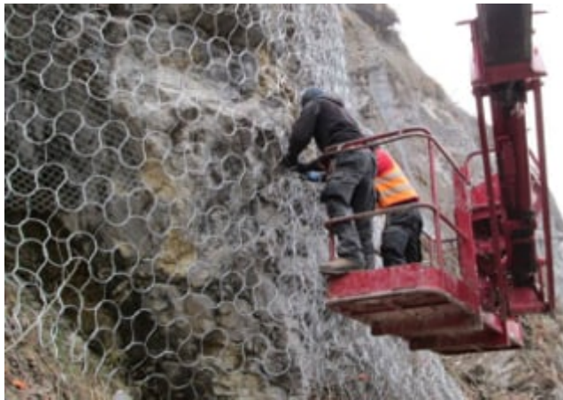
Installation of Omega-Net for slope stabilization.
