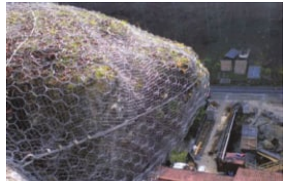
Heavy rock stabilization using Omega-Net.
