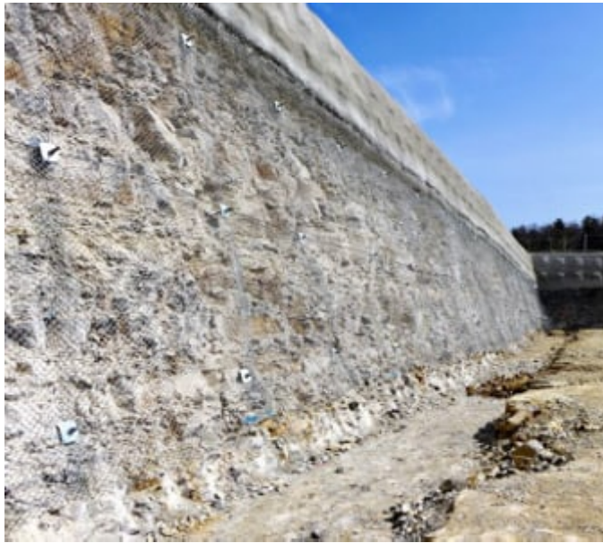
Rock wall reinforced using High Performance Netting.
