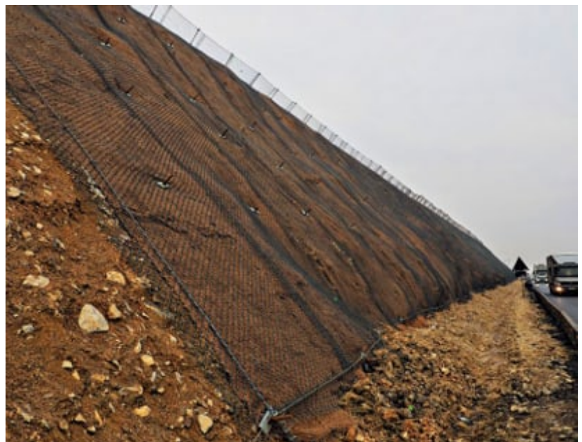
The use of HPN+ in combination with organic mats greatly reduces the lost of fine material and encourages revegetation.
