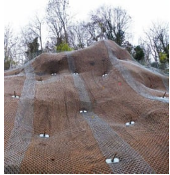
Anchored mesh system (slope retention system) using a high tensile mesh and anchor system based on loading conditions.
