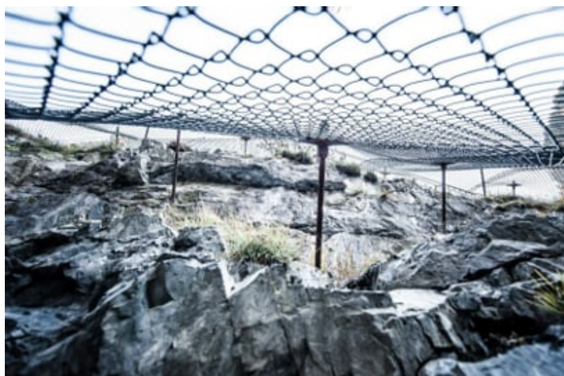
An example of a slope mesh system designed to protect a highway from falling ice that builds up on the slopes during the winter.
