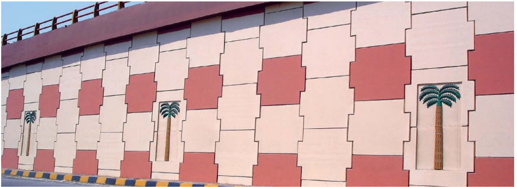
Navghar Flyover, Mumbai International Airport Mumbai, India ►
