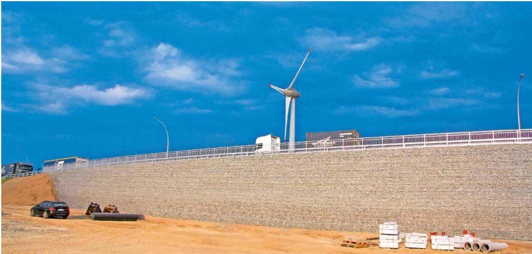
Retaining Walls in Altenwerder
