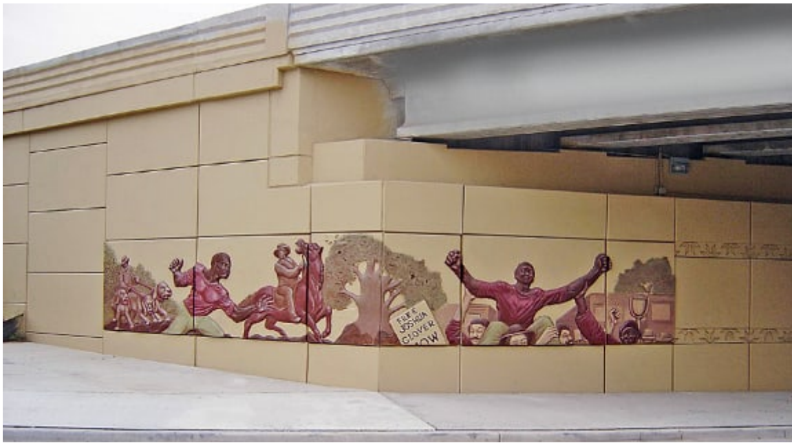
Marquette Interchange Milwaukee, Wisconsin, USA ►
