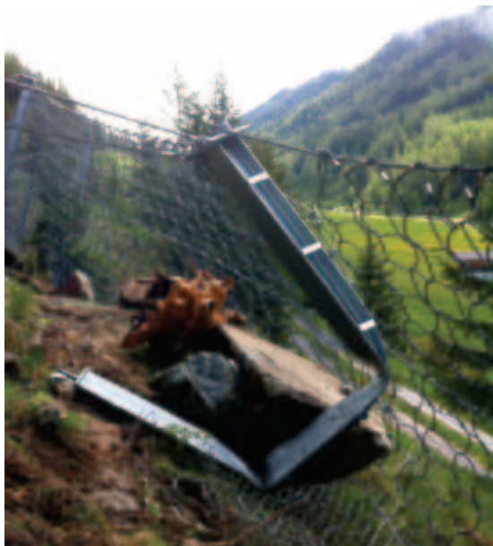
Two examples of hinged rockfall catchment fences impacted at and surrounding a post. Posts by Trumer are robust and can withstand direct impacts without compromising the systems integrity.
